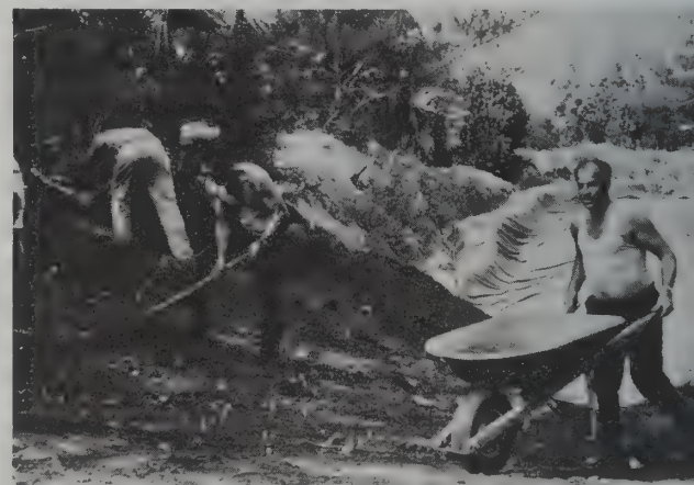
Constructing the artificial freshwater pond, 1975.
